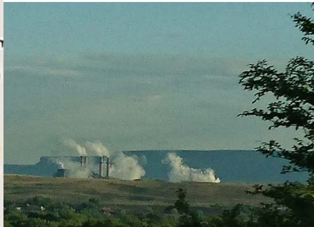
Four Corners Power Plant
